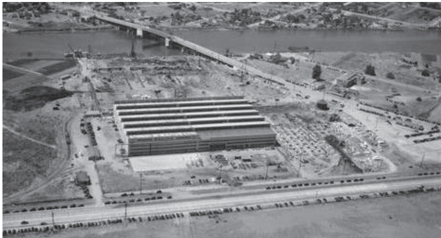
NOW YOU SEE IT: Boeing plant with tell-tale saw tooth roof later disguised as a fake town called Wonderland – USAAF, National Archives
